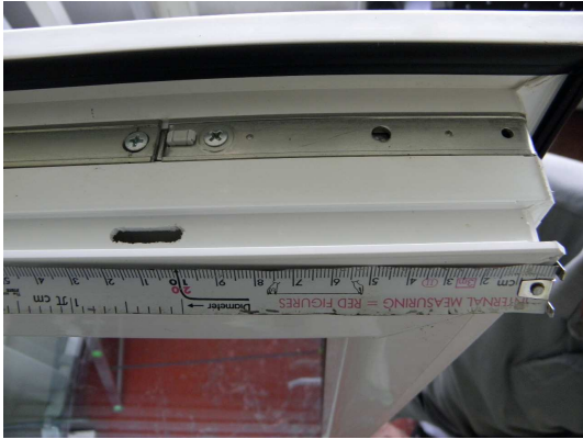
Picture 25 Vapour pressure equalisation
