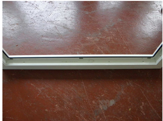
Picture 22 View of horizontal glazing rebate
