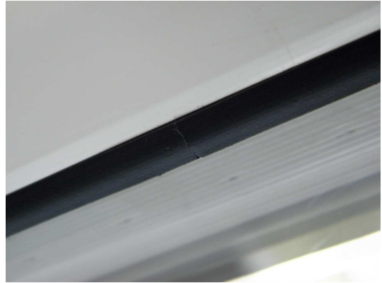
Picture 20 External glazing seal, sealant joint
