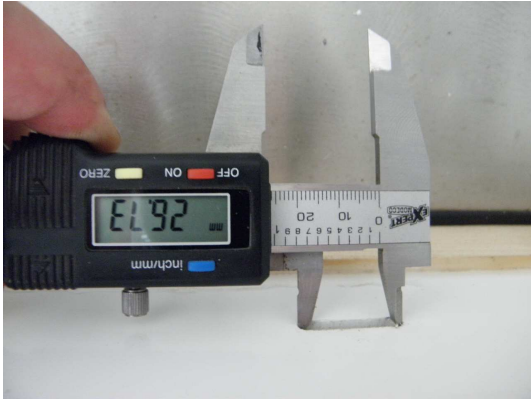
Picture 7 Rebate drainage
