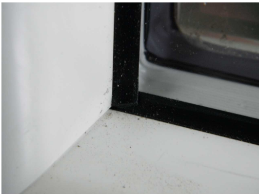
Picture 23 Internal glazing seal, corner configuration
