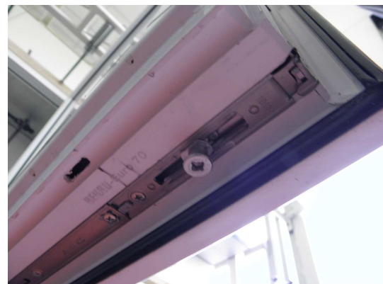
Picture 36 Locking situation, frame member / casement member 3
