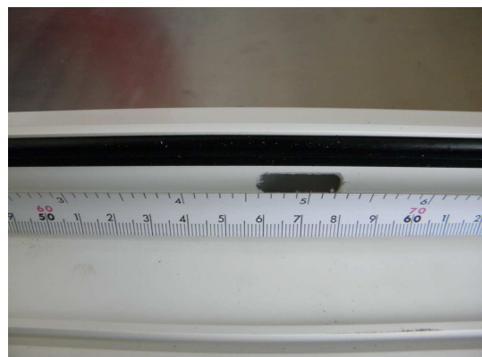
Picture 6 Rebate drainage
