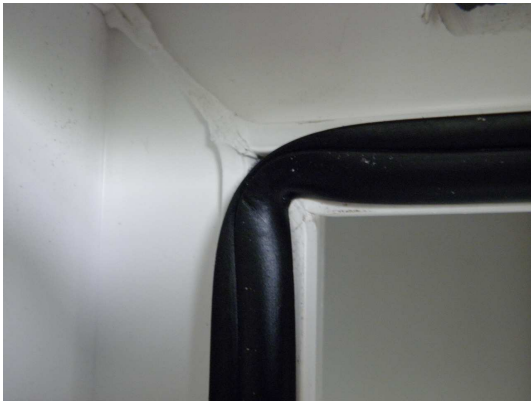
Picture 9 External rebate seal, corner configuration
