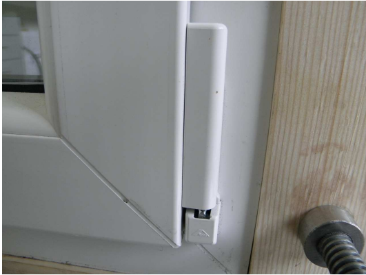
Picture 31 Corner pivot, internal view
