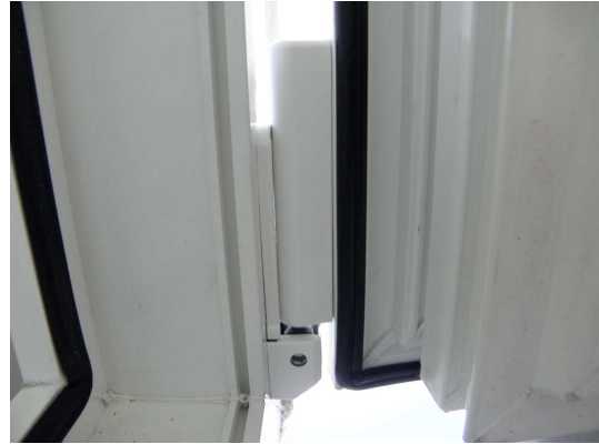
Picture 32 Corner pivot, rebate view
