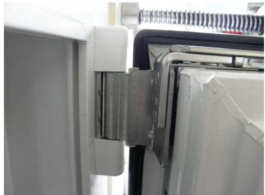
Picture 30 Tilt mechanism pivot, rebate view
