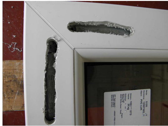
Picture 38 Cutback reinforcement casement member
