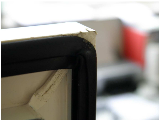
Picture 11 Internal rebate seal, corner configuration
