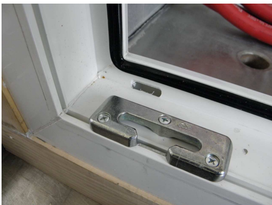
Picture 35 Locking situation, frame member / casement member 3
