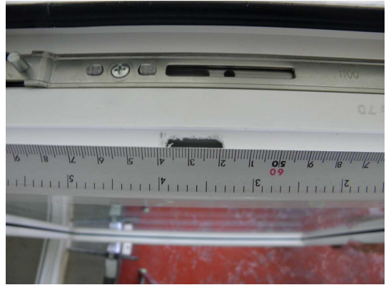
Picture 26 Vapour pressure equalisation
