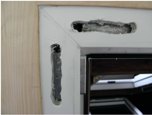
Picture 37 Cutback reinforcement frame member
